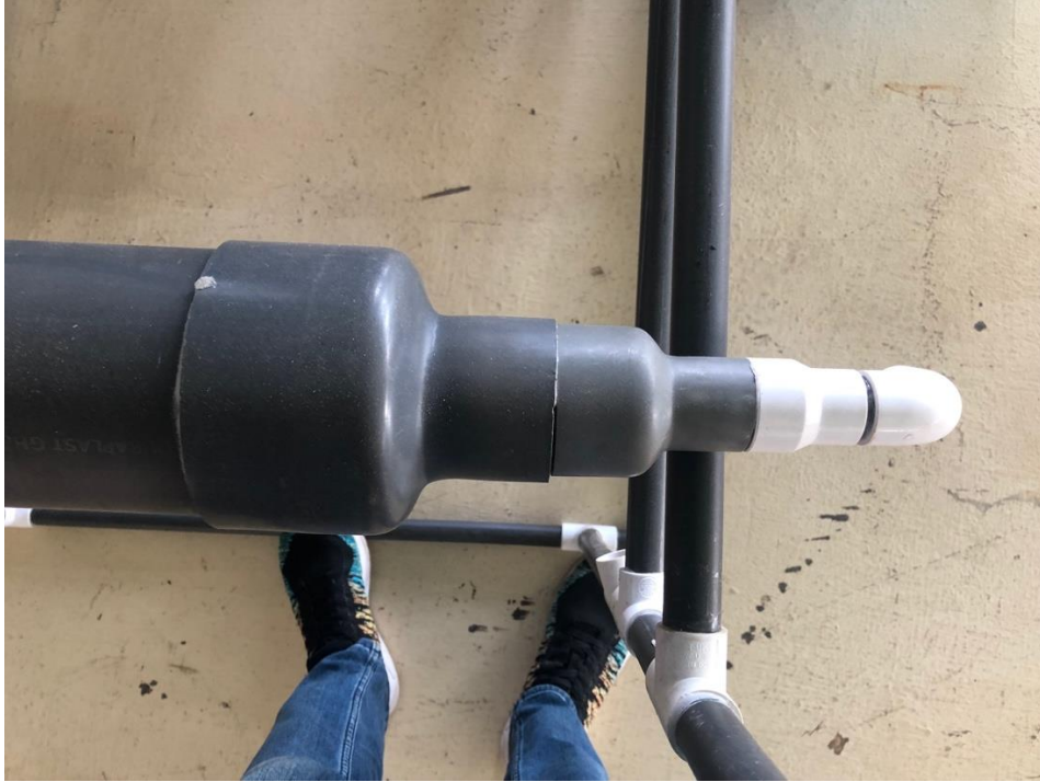
Figure 5. Reducing the 4-inch pipe to 3/4-inches
