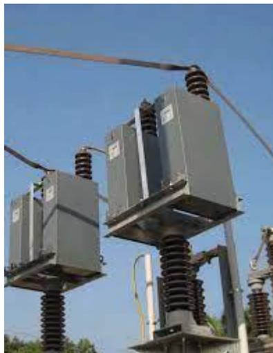
Figure 3.3: Voltage Transformer
