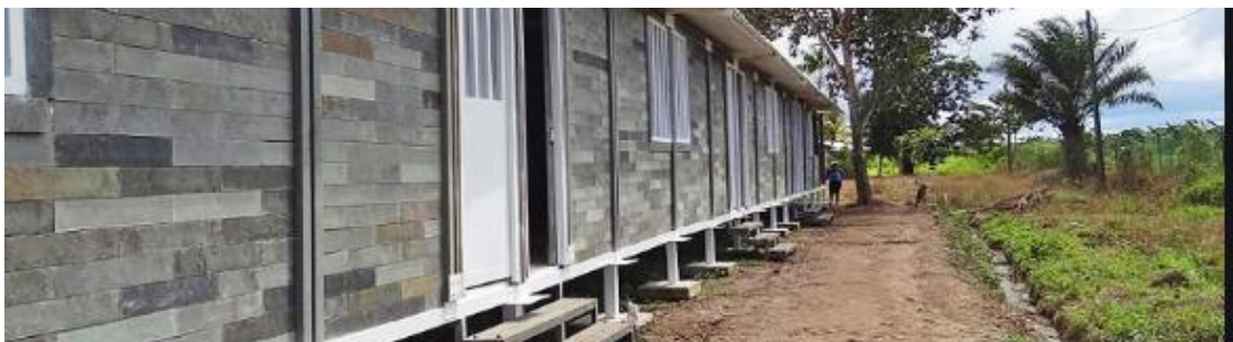
Figure 2: Picture of a house made out of plastic bricks (Conceptos Plasticos, 2016)
